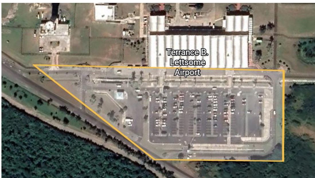
Figure 1 Parking lot at the Terrance B. Lettsome International Airport.
